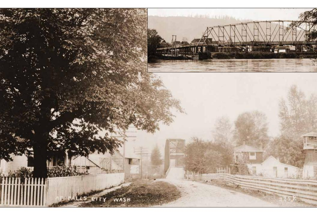
The first Snoqualmie River bridge at Fall City was a wooden bridge, 350 feet long and 16 feet wide, completed in 1889. It fell without warning in the spring of 1900. The materials were salvaged and it was rebuilt in 1901. In 1908, steel beams were added to make it stronger, but it was then replaced in 1917 with a concrete bridge due to greatly increased traffic levels.
